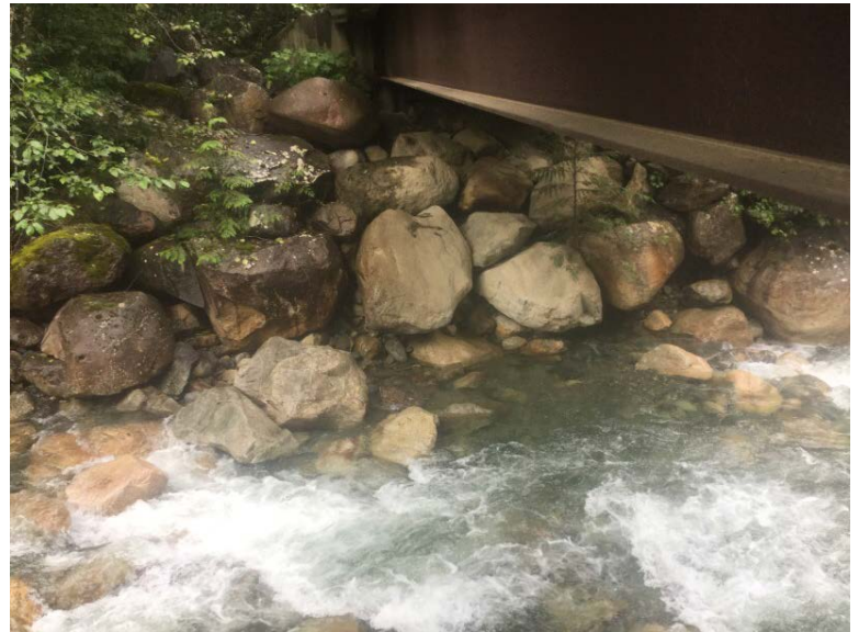
Left Bank Abutment when facing downstream
