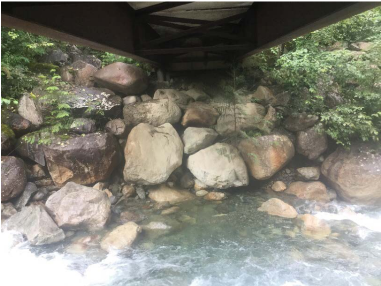
Left Bank Abutment when facing downstream
